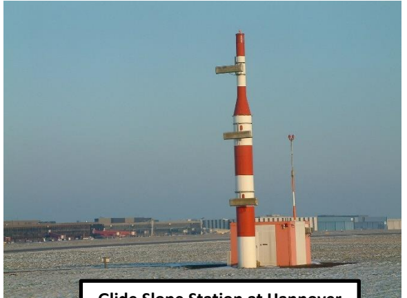
Glide Slope Station at Hannover
